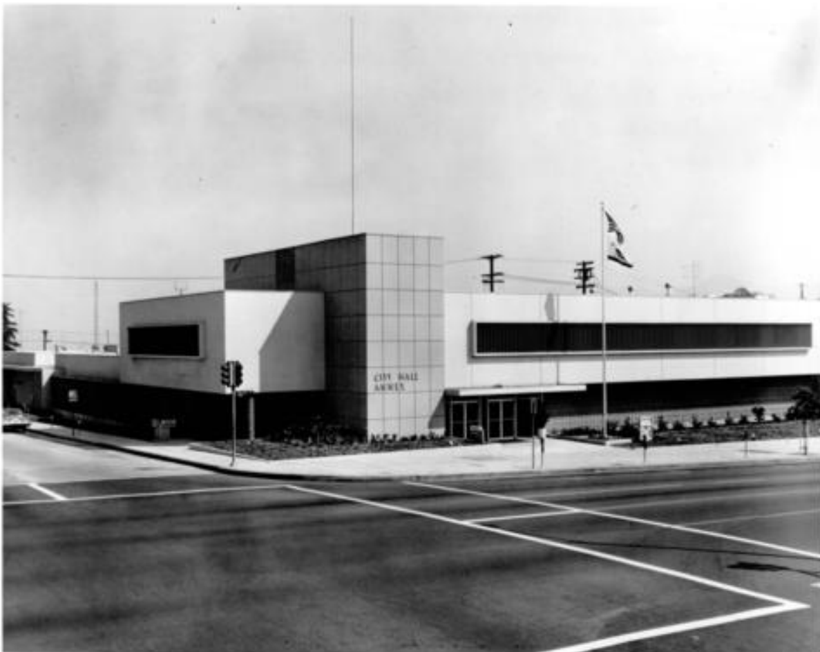
Burbank Civic Center Annex at 250 E. Olive Avenue, Burbank. Designed by Prescott and Whalley, 1959 (extant). Circa 1960s. Source: Burbank Public Library, Burbank in Focus.
