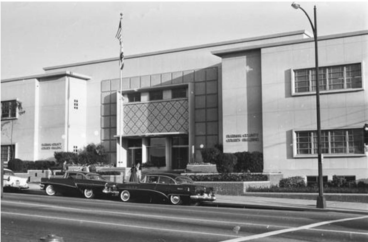
Burbank County Courts Building at 300 E. Olive, Burbank. Designed by Prescott and Whalley in 1954 (extant). Circa 1950s. Source: Burbank Public Library, Burbank in Focus.
