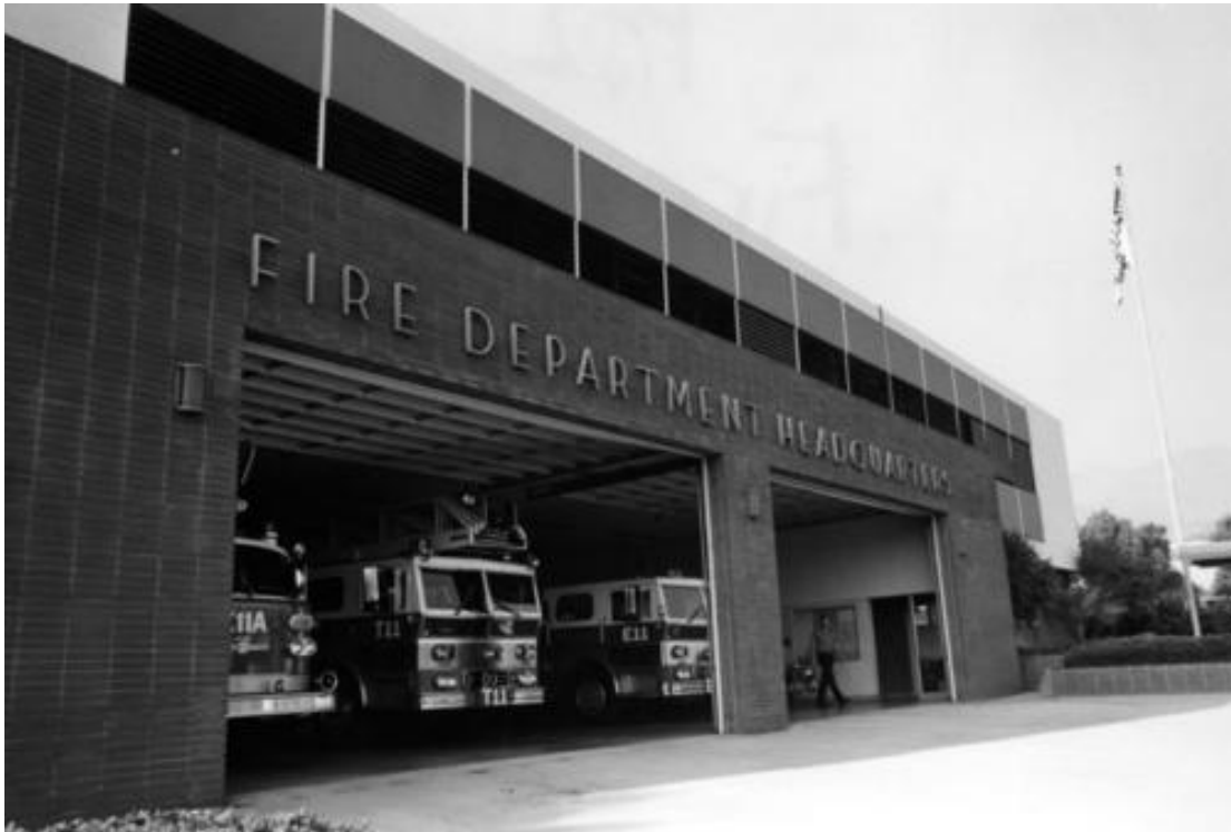
Main Headquarters Fire Station Burbank at 353 E. Olive, Burbank. Designed by Prescott and Whalley in 1961 (not extant). Source: Burbank Public Library, Burbank in Focus.
