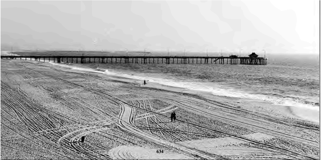
View from third story, facing southwest, 1969. Source: Our Lifeguard Family .
