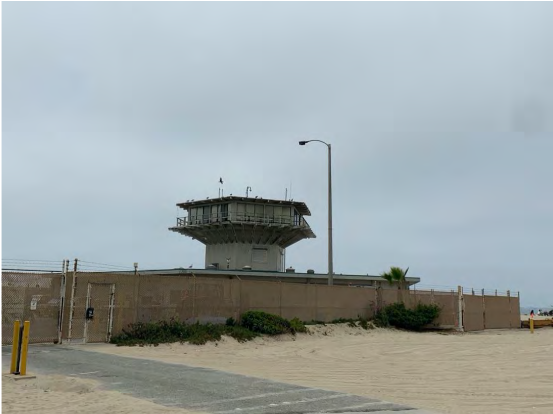
View facing northwest, 2023.
